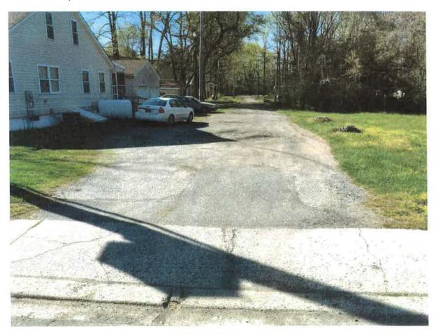
Conwell St. currently consists of over 34 pot-wholes and is about 12' feet wide and over 400' feet long. Conwell St. is in deplorable condition, which through the years has caused community members to obtain wheel-alignment services and new tires due to the rapid decline in the conditions of Conwell St.
